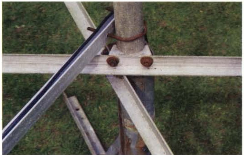
● Fig. 4: Method of fixing the element supports and the coaxial cable support to the mast.
